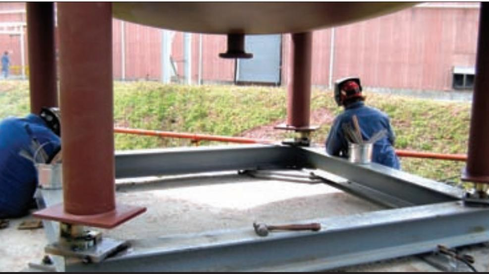
Install with care: Pictured is a compression load point installation on a four-legged vessel. Four legs offer a larger area to support the vessel, provide for equal load sharing among the legs, and help to keep the vessel from tipping over.
